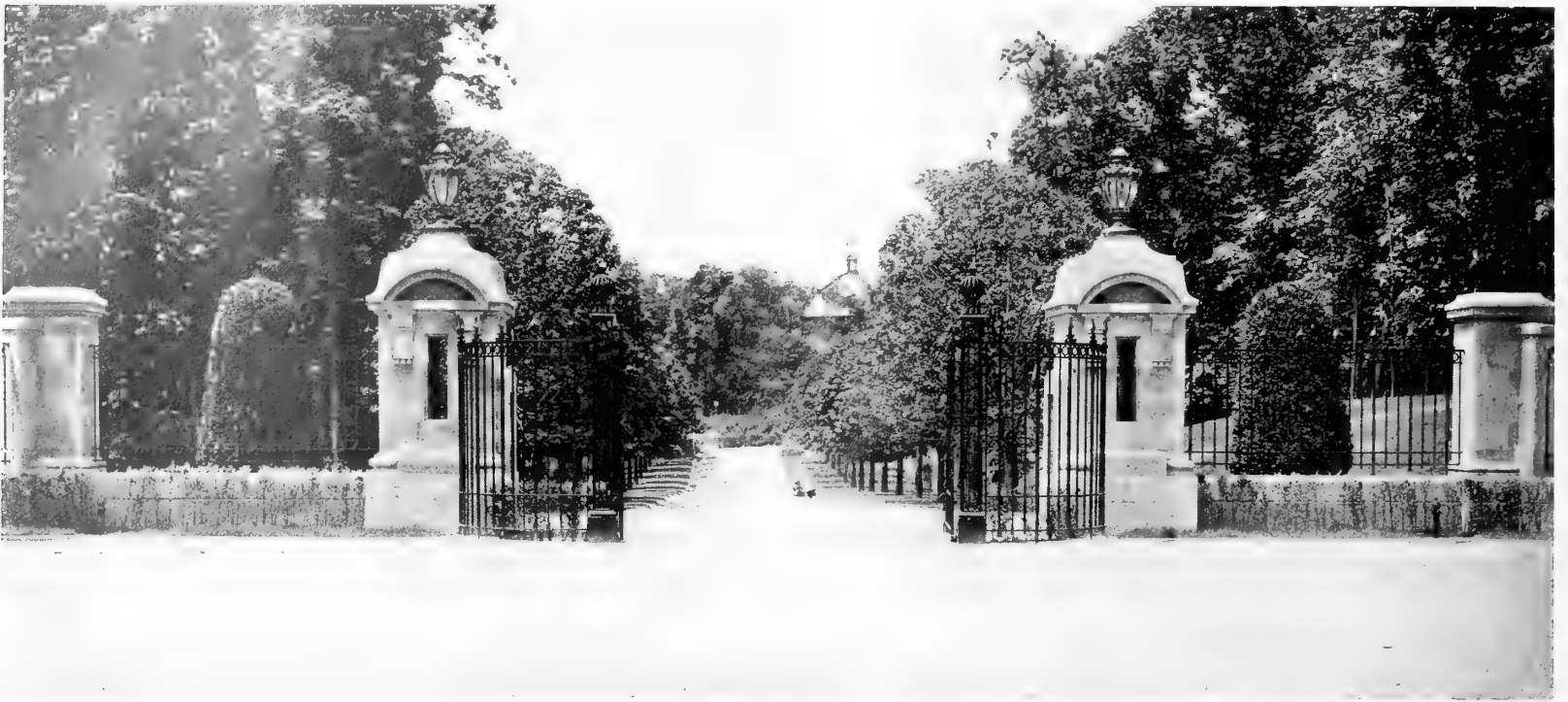
The Entrance Should Be Wide Enough for Two Vehicles to Pass Each Other
